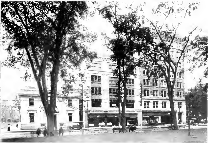
WEST MAIN STREET ARCHITECTURE, WATERBURY From left to right: Colonial Trust Company; Hampson and Lilley Buildings. Viewed from the green.
